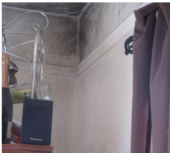
Photograph 2: Damp and mould hazard
